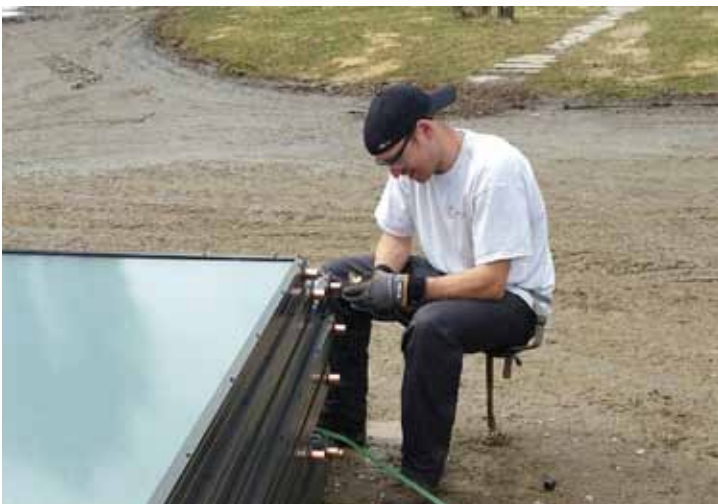
Hamley Farms | Barton, NY | Assembly & Installation
